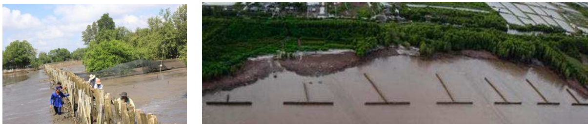
Fig. 20 Wood or bamboo fences protect against waves and favour natural regeneration (source: vietnamnews.vn 2015, Schmidt and Duke, 2016)
